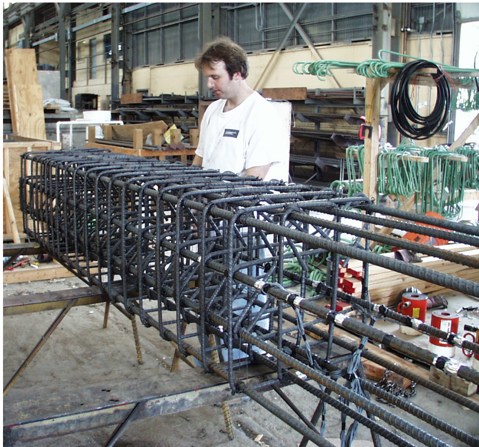
Figure 3.8 Construction of Column Cage
