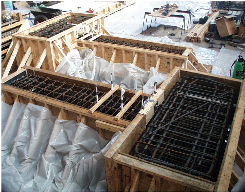
Figure 3.6 Formwork before Concrete Casting
